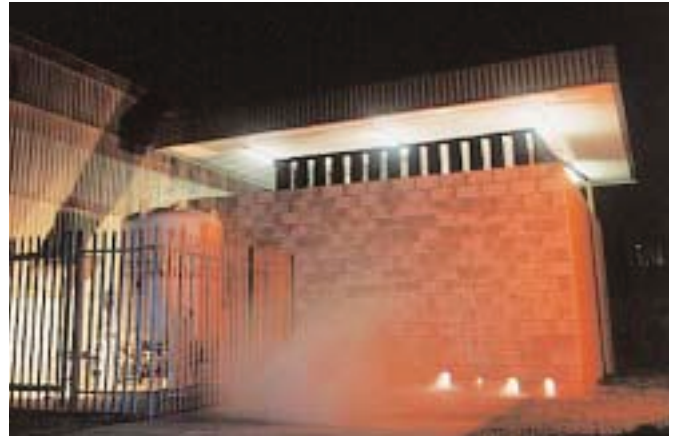
Cryogenic Test Facility/Explosion Proof Chamber.
